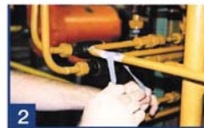
remove paint and clean pipe
