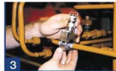
clamp SC onto pipe
